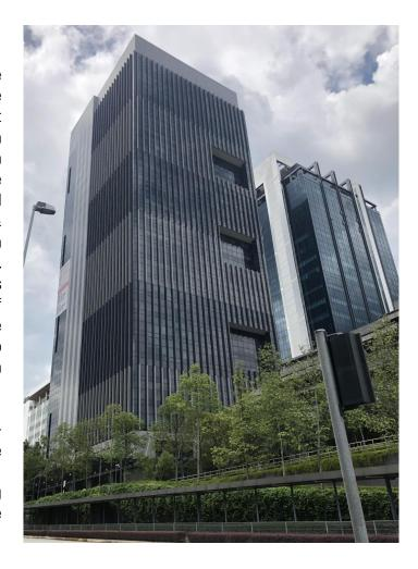
Having planned from its initial stage of going green and coupled with an MSC status, much emphasis was employed in its passive design initiatives and balanced by its active components to make it an Energy Efficient building. High efficiency glazing with double glazed 12.88mm glass, gives the advantage of low E with superb performance and durability assured.
