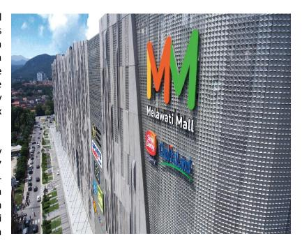
This is enhanced by the façade performing an Overall Thermal Transfer Value (OTTV) of the building as low as  $32.2 \text{ W/m}^2$  for its building envelope as compared to the Malaysia minimum standard of  $50 \text{ W/m}^2$ .
