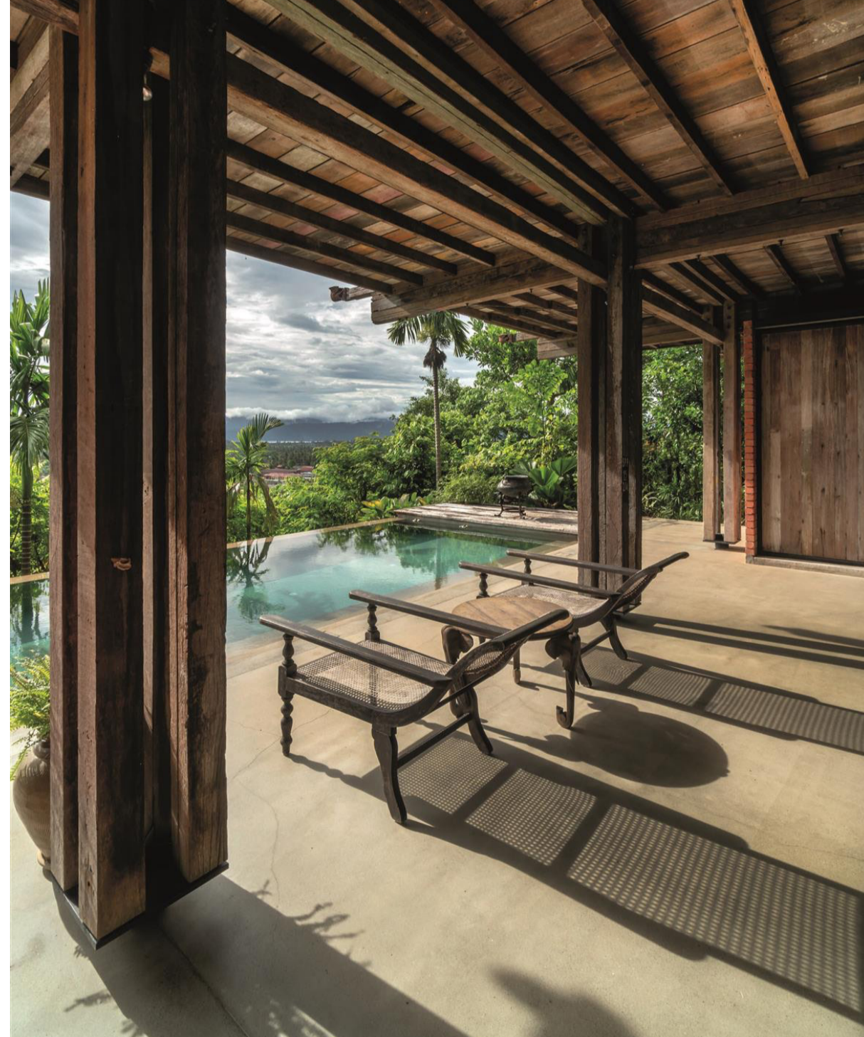
The Telegraph Pole House in Langkawi is constructed using old telegraph poles found in a timber yard in Alor Setar.
