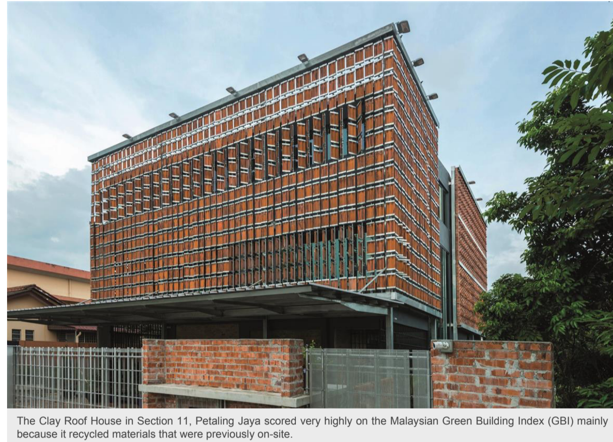
The Clay Roof House in Section 11, Petaling Jaya scored very highly on the Malaysian Green Building Index (GBI) mainly because it recycled materials that were previously on-site.
