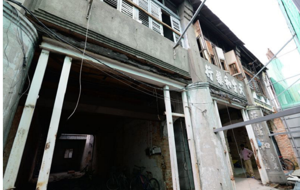
The frontage of the five shophouses along Kimberley Street.
