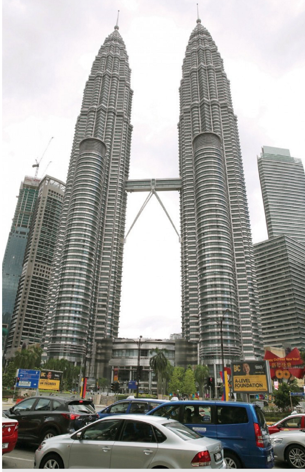
Despite being surrounded by new office buildings, Petronas Twin Towers is still the most wanted address for many MNCs. (Photos by The Edge)
