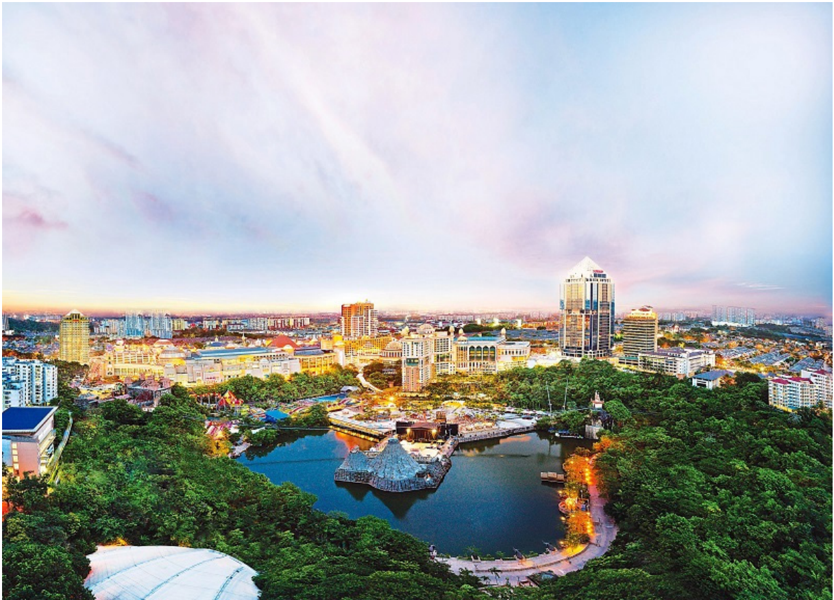
Sunway Resort City, the nation's first Green Building Index (GBI) certified green township.
