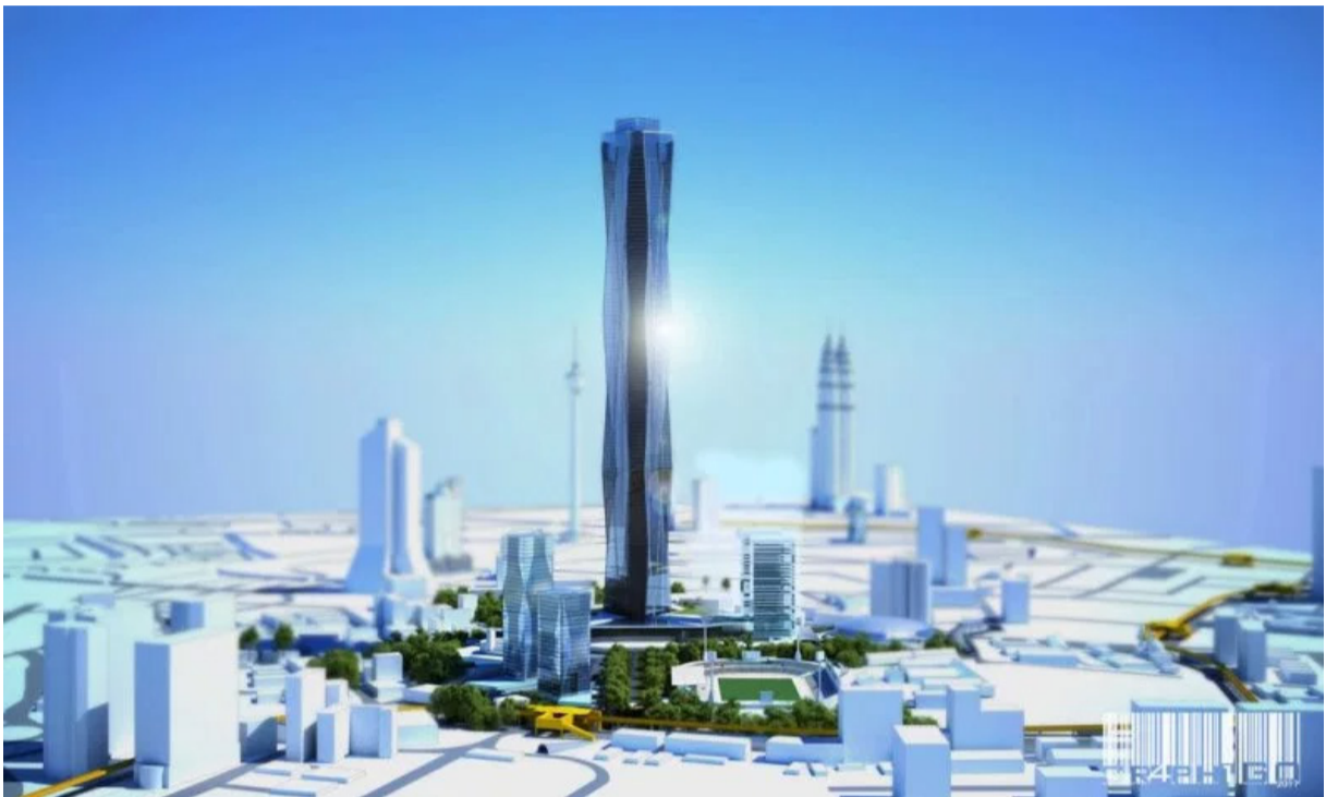
The 118-story tower will become a new iconic feature of Kuala Lumpur's skyline. Photo Credit: PNB
