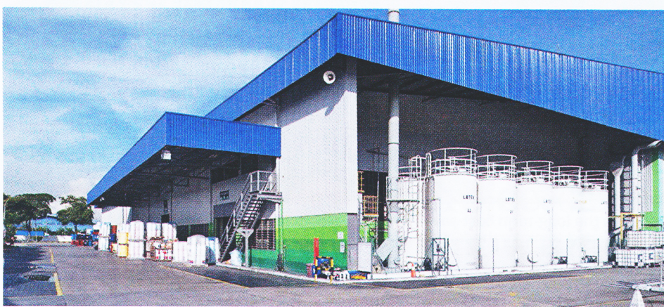
Nippon Paint's manufacturing facility in Shah Alam
