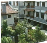
External façade shading to reduce solar heat gain and lush greenery to reduce heat island effect
