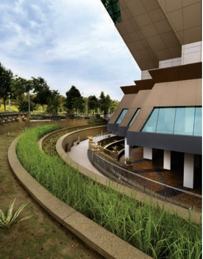
Landscaping surrounding the building helps reduce the urban heat island effect. On-site composting provides nutrients for plants, reduces the need for fertilizers and reduces waste.
