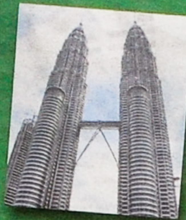
The country's iconic Petronas Twin Towers would not be what it is without high performance glazing.
